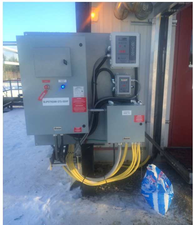
SlipStream® GTS-DeHy supervisory control panel plate complete with main BMS and aux BMS
