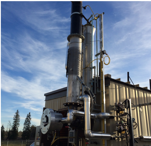
SlipStream® GTS-DeHy glycol reboiler building showing new main burner and aux burner assemblies
